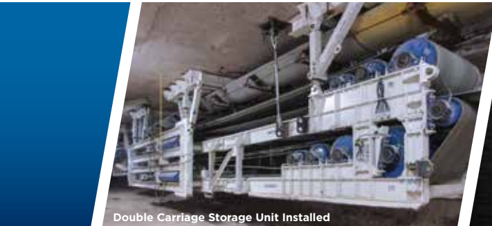
Double Carriage Storage Unit Installed
