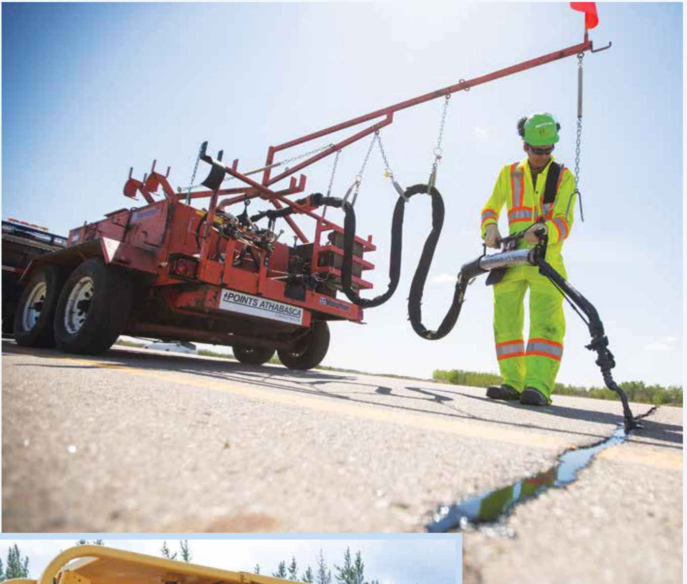
Highway 11 crack sealing project.
