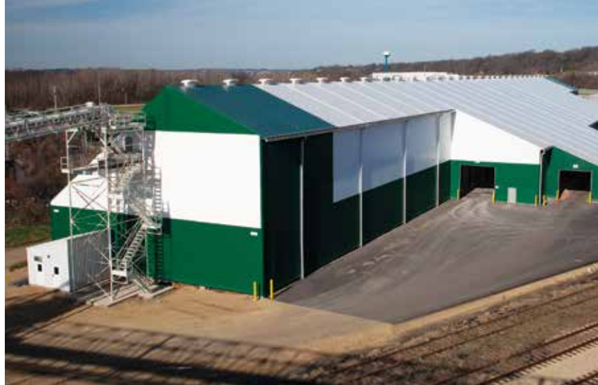
IEI Barge, East Dubuque, IL.
